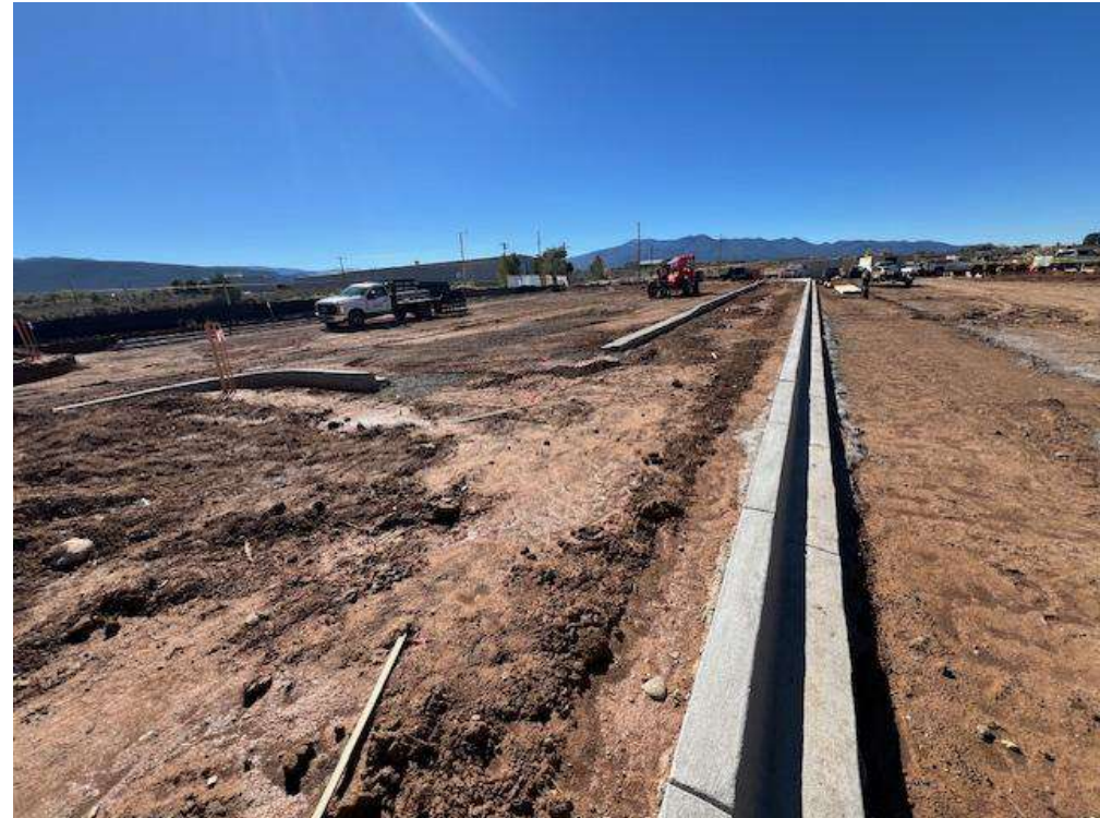
Curb and Gutter / Grading
