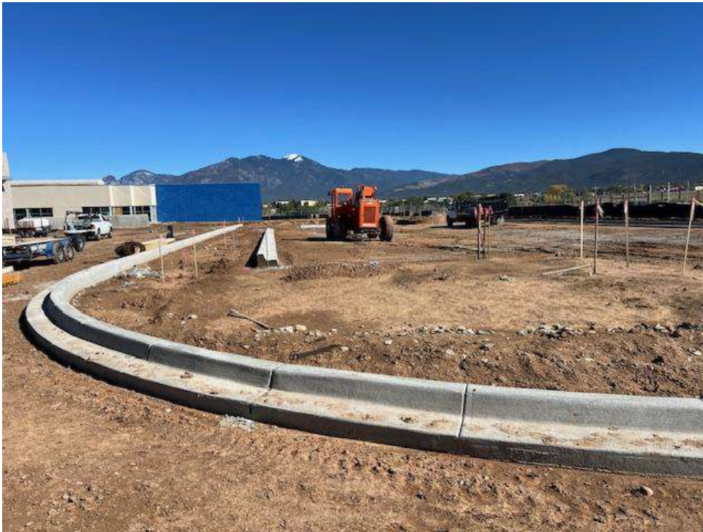
Curb and Gutter / Grading
