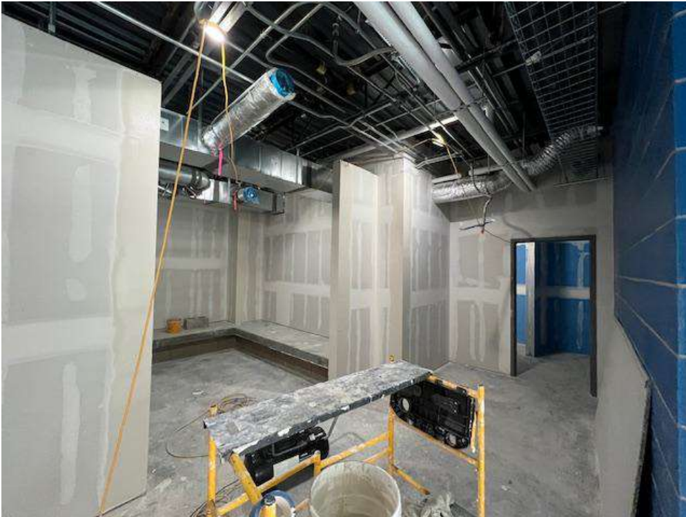
Sheetrock Rough In
