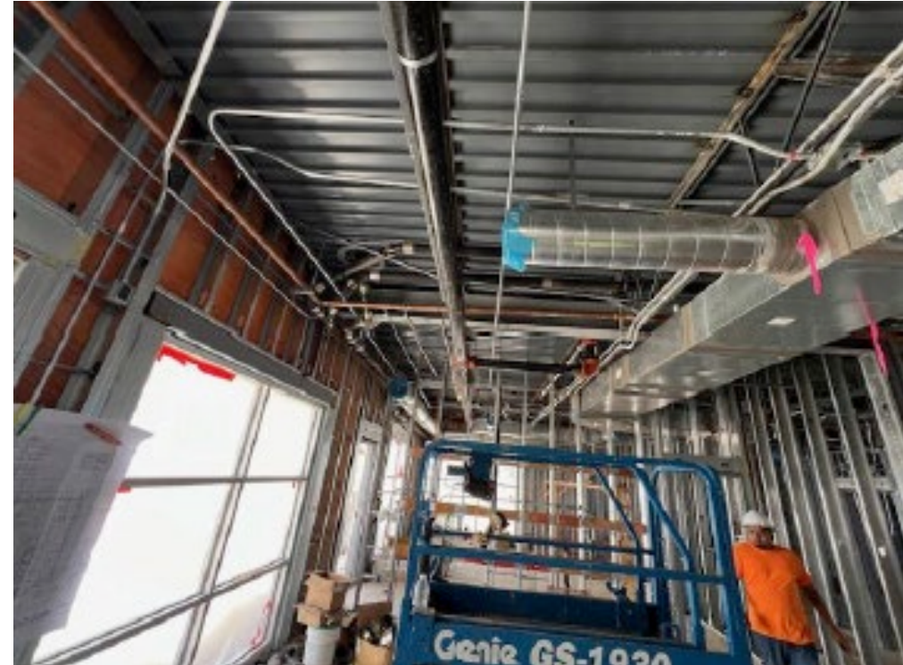
MEP Rough-in / Windows / Wall Framing
