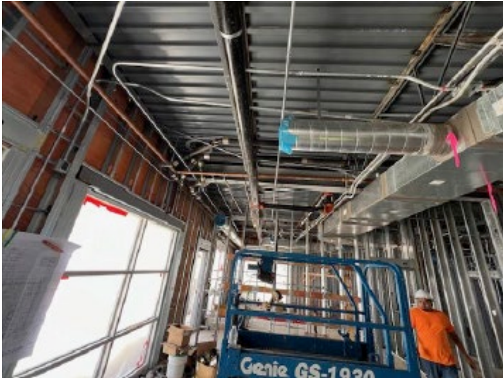
Mechanical, Electrical, Plumbing Rough In
