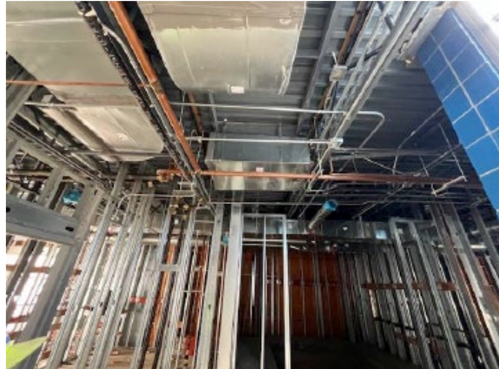
Mechanical, Electrical, Plumbing Rough In
