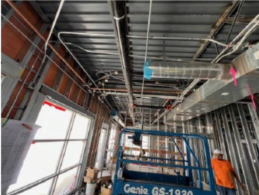
Mechanical, Electrical, Plumbing Rough In
