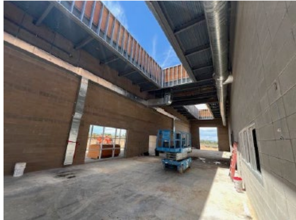
Mechanical, Electrical, Plumbing Rough In
