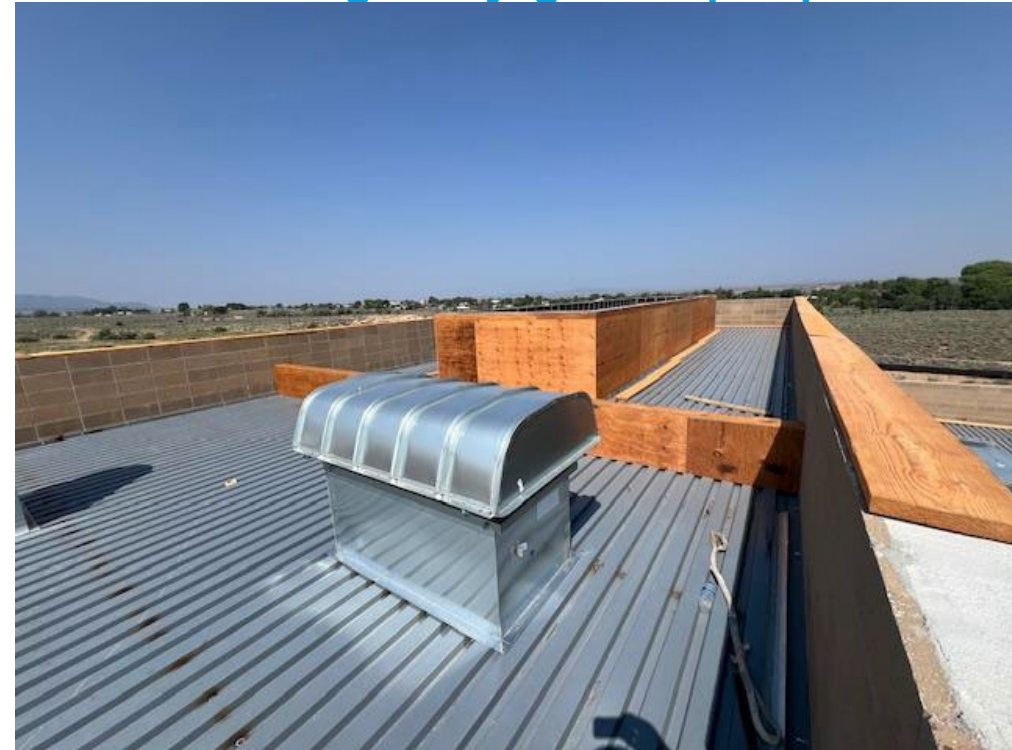
Exhaust fan, metal deck & plywood sheathing at skylight and parapet
