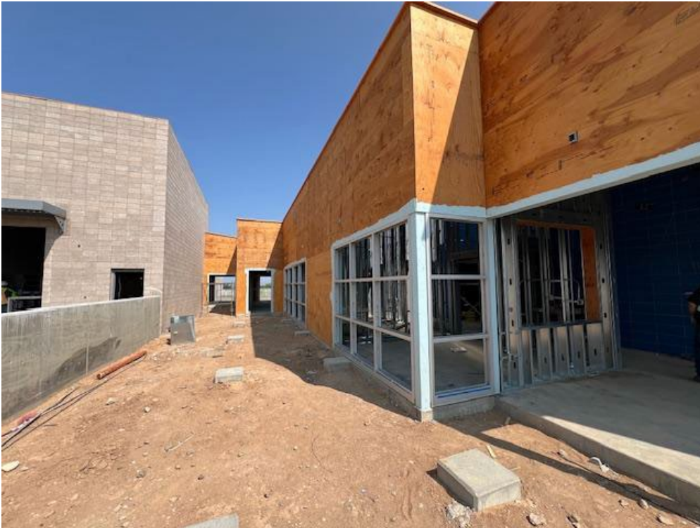
Plywood sheathing & aluminum storefront installation
