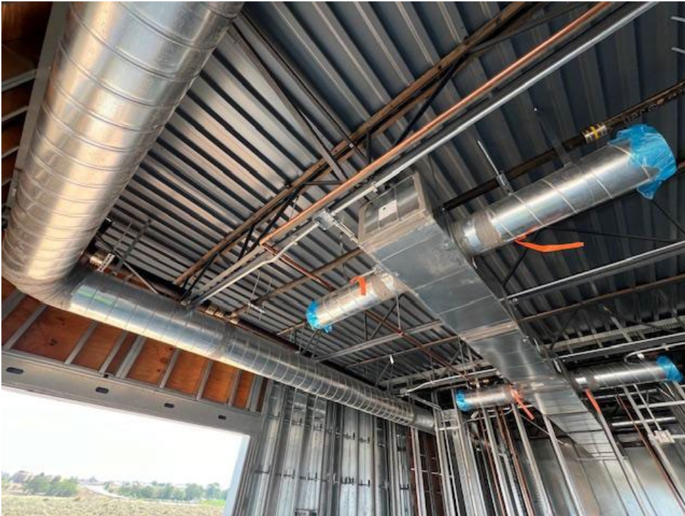
Steel studs & plywood sheathing
