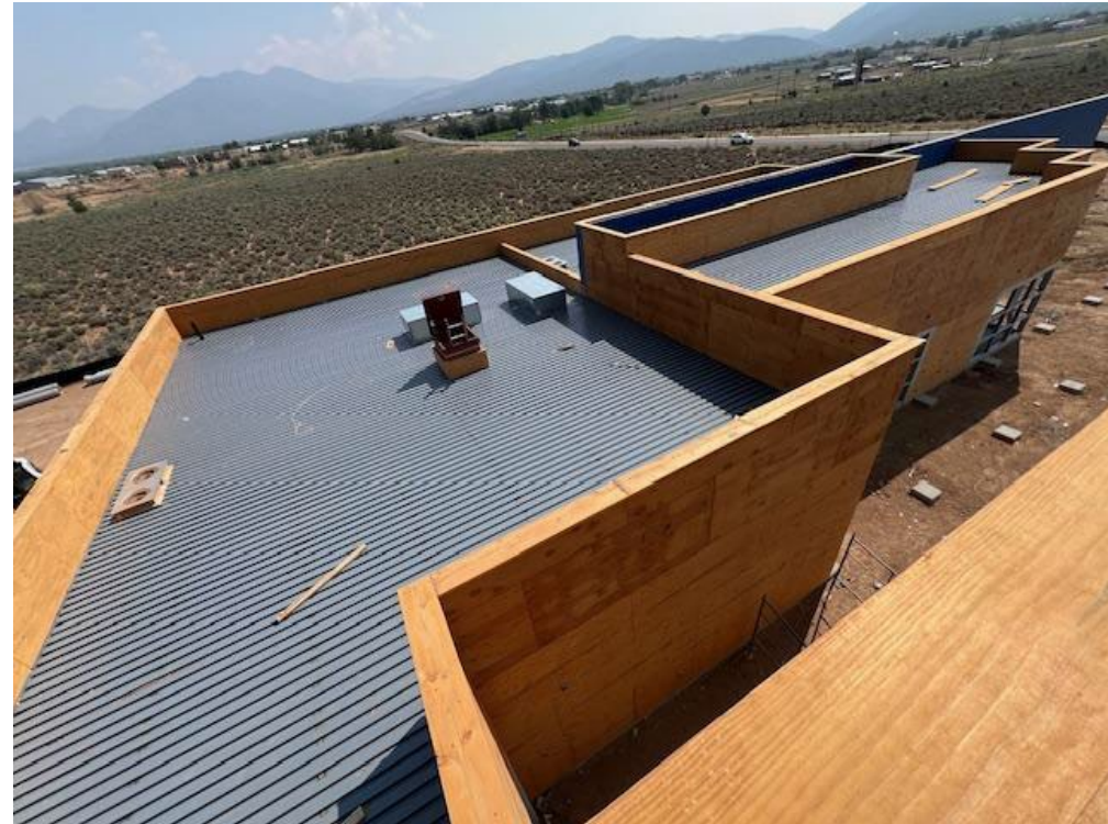
Plywood sheathing and roof access
