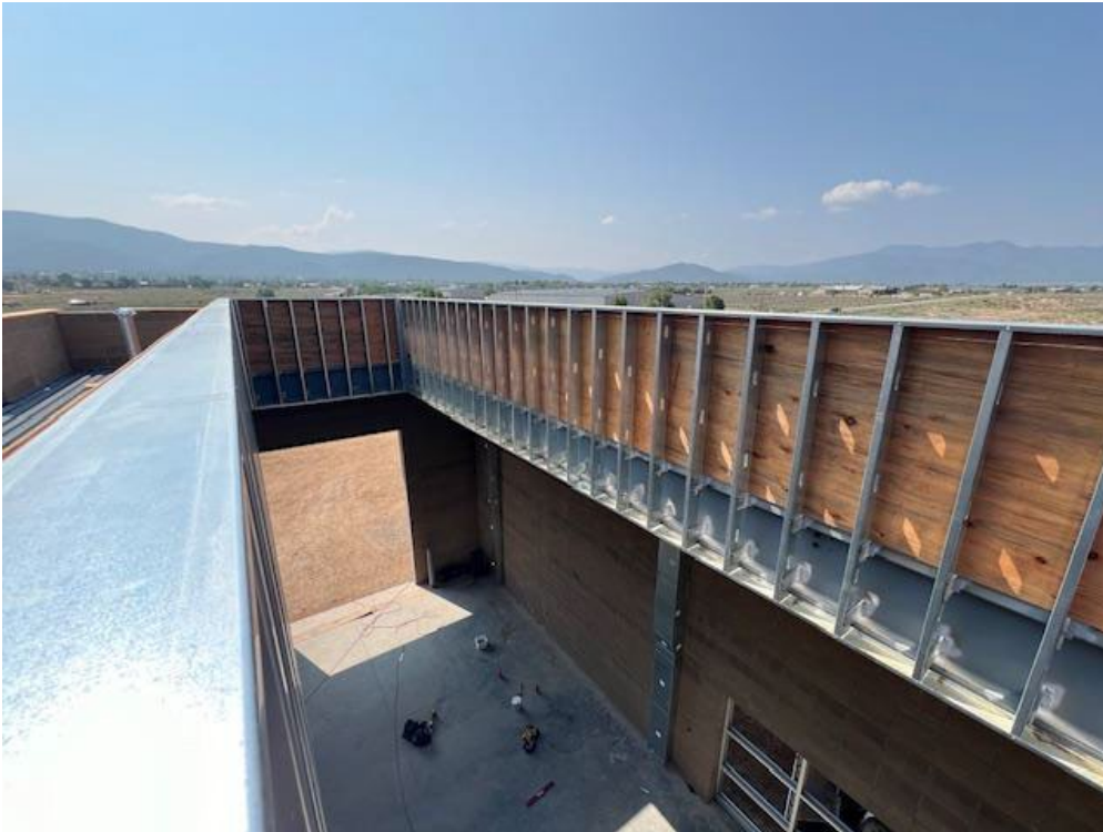
Bus bay skylight
