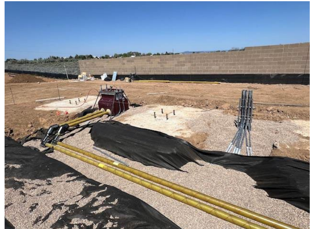
Fuel island gravel backfill and footings
