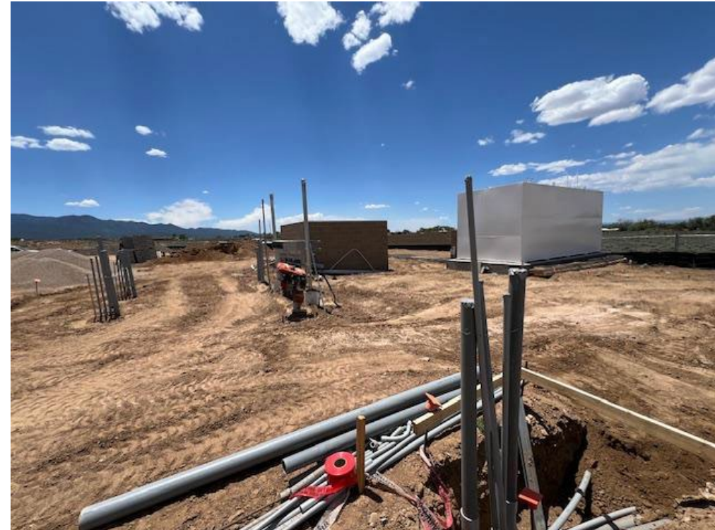
Electrical rough-in at generator pad
