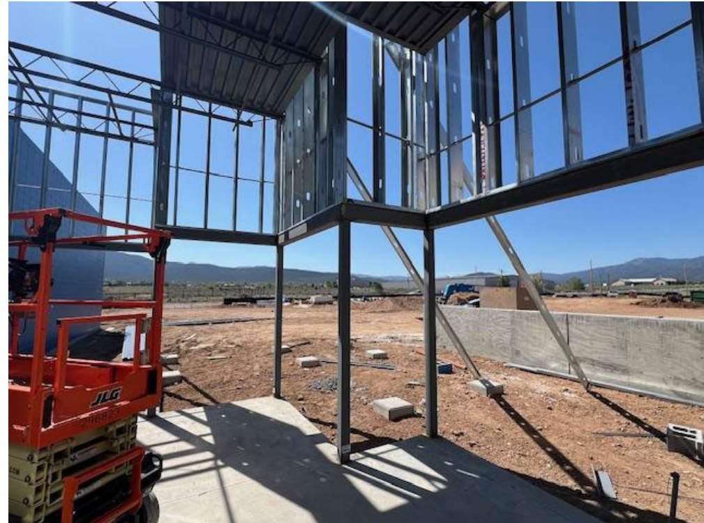
Front entry steel erection
