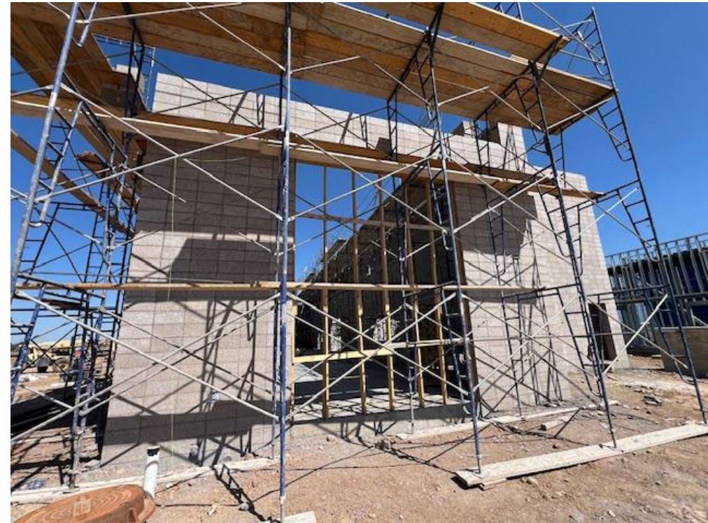
Wall erection at but bay
