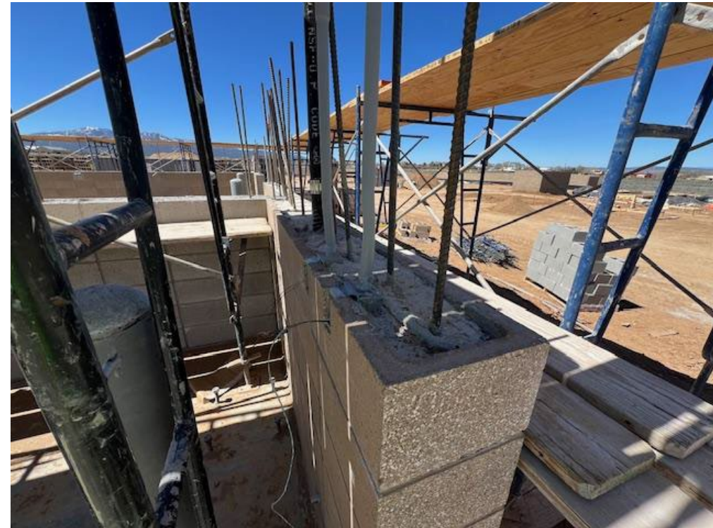
Wall, rebar and electrical conduit
