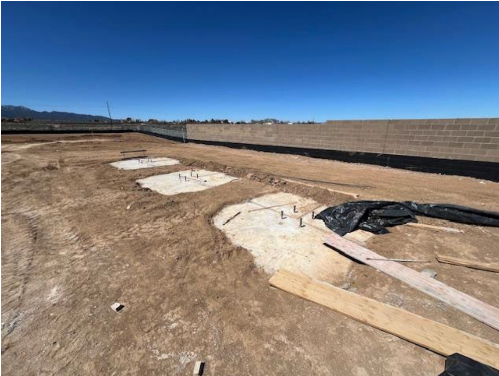
Footings and embeds for canopy
