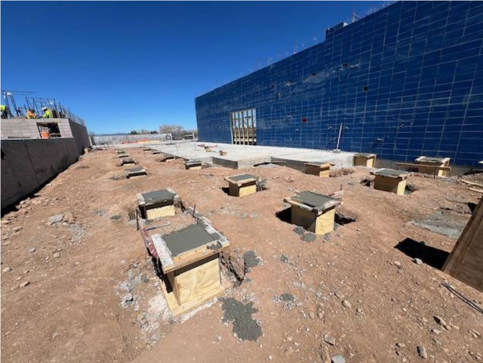
Blue spin wall and column footings
