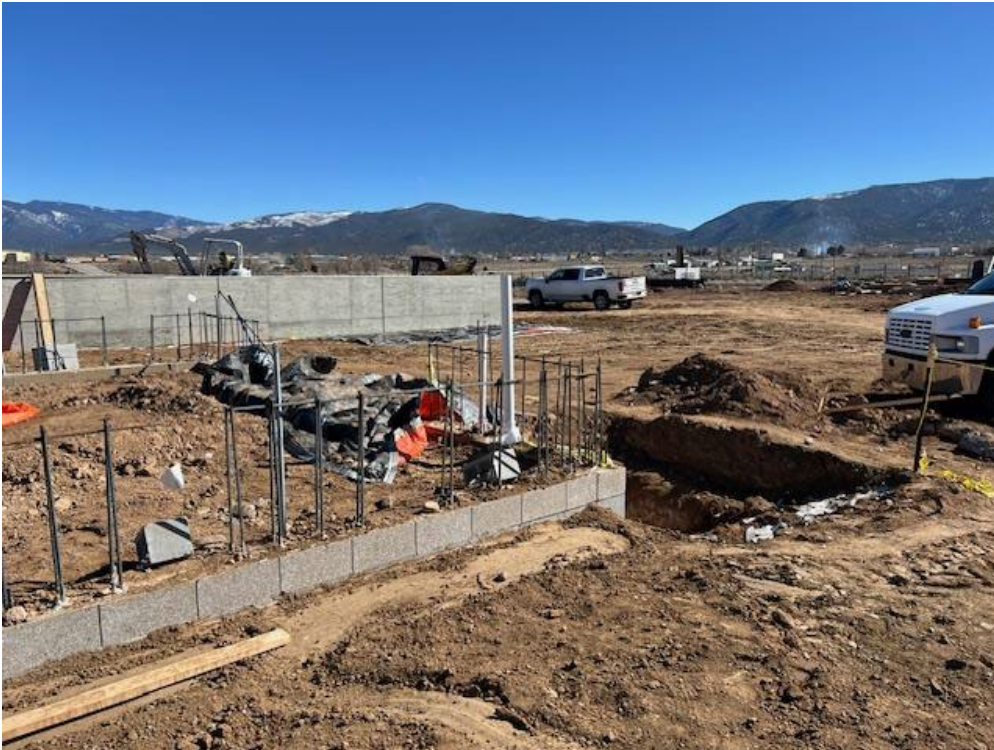
Concrete masonry, rebar, plumbing, electrical
