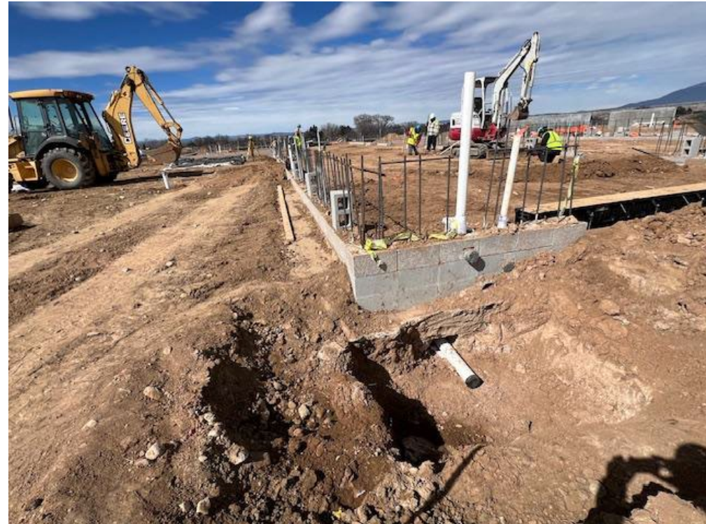
Stem wall, electrical conduit, plumbing
