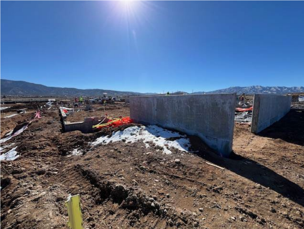
Concrete wall at outdoor patio courtyard
