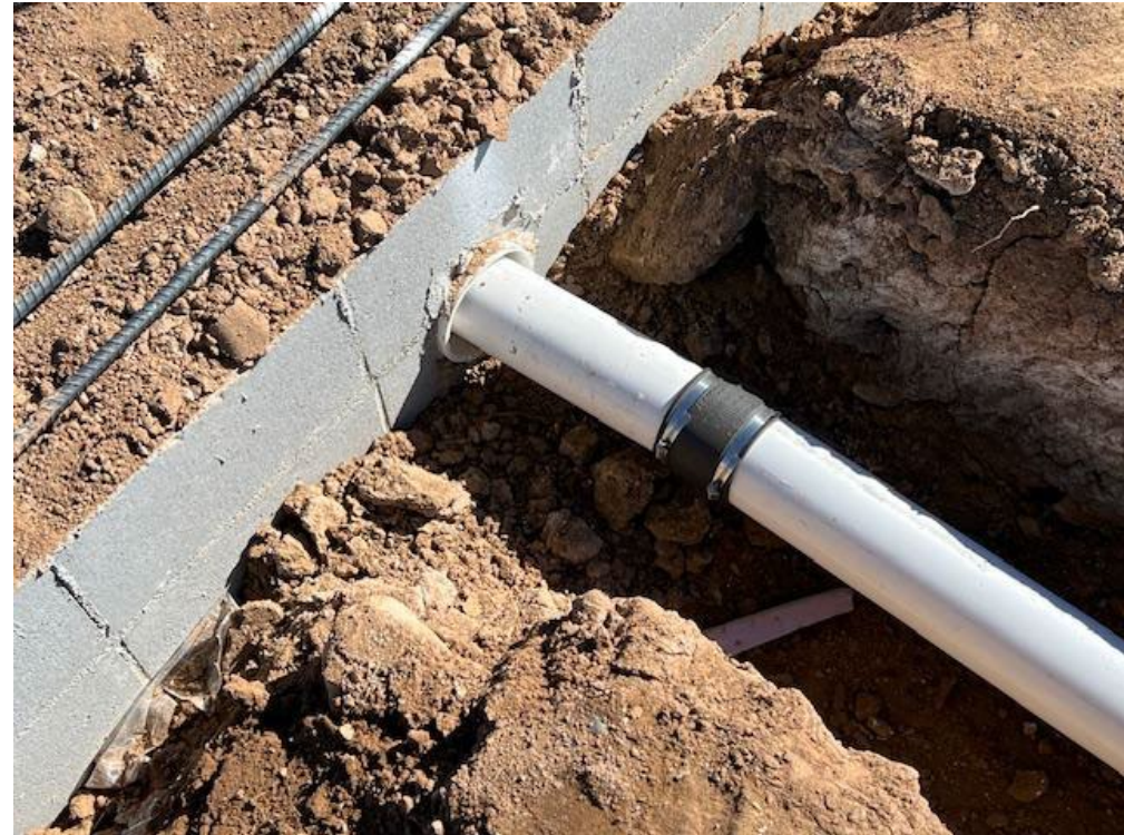
Plumbing through stem wall
