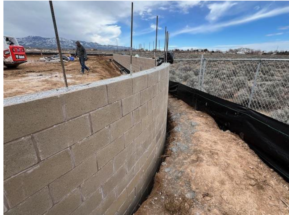
Retaining wall grouted
