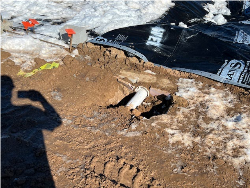
Plumbing penetration at stem wall
