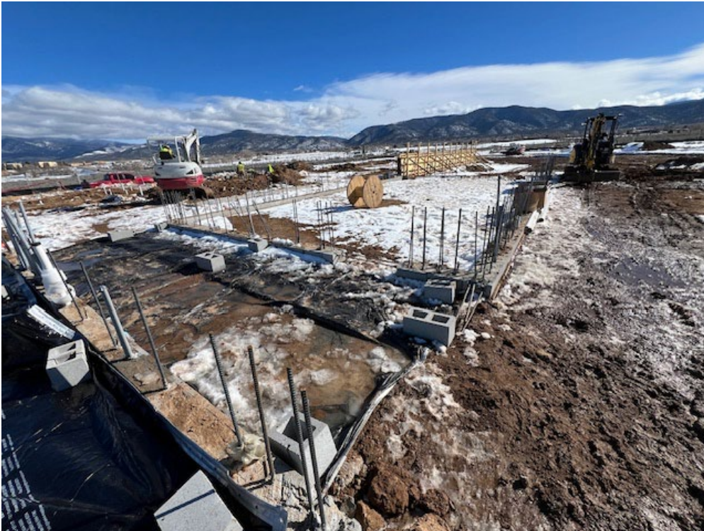
Protective blankets, stem walls, rebar
