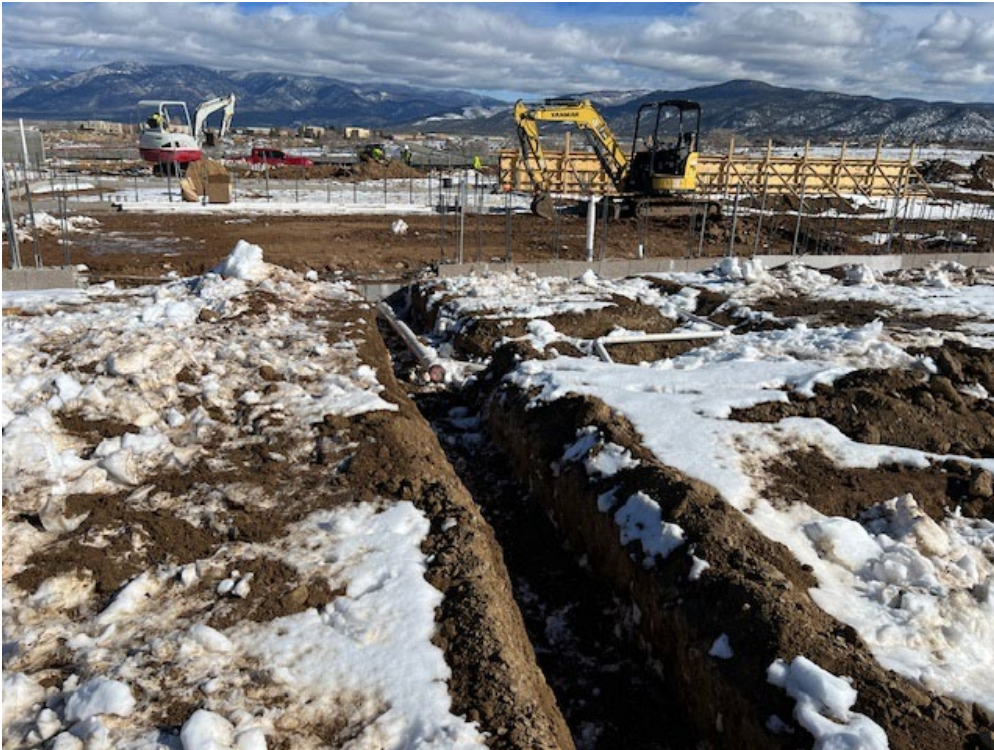
Underground plumbing and trench
