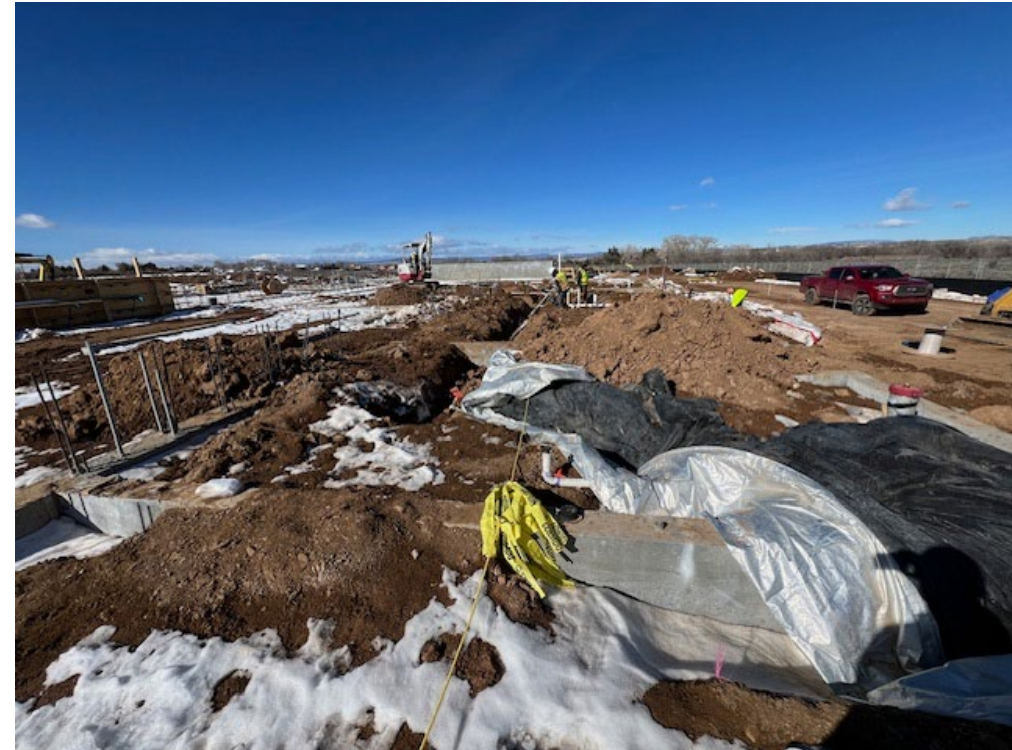
Stem walls, conduit, plumbing
