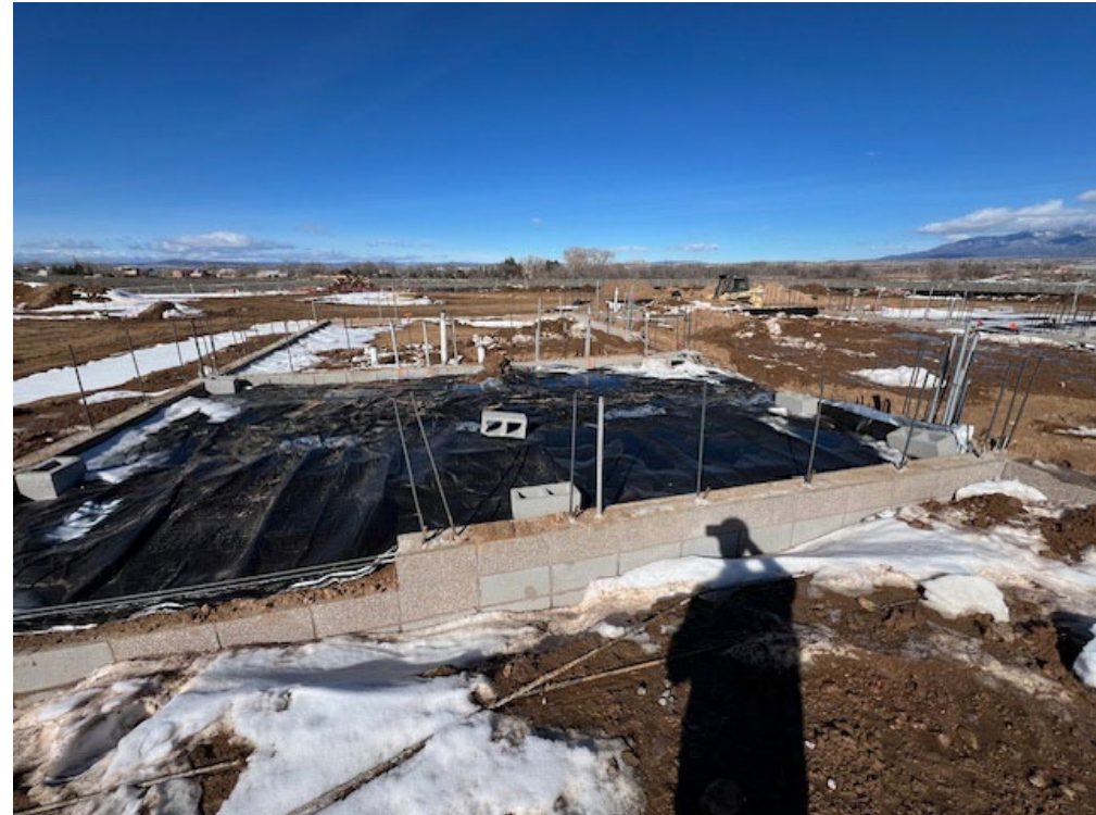
Cinder block stem wall with rebar and conduit
