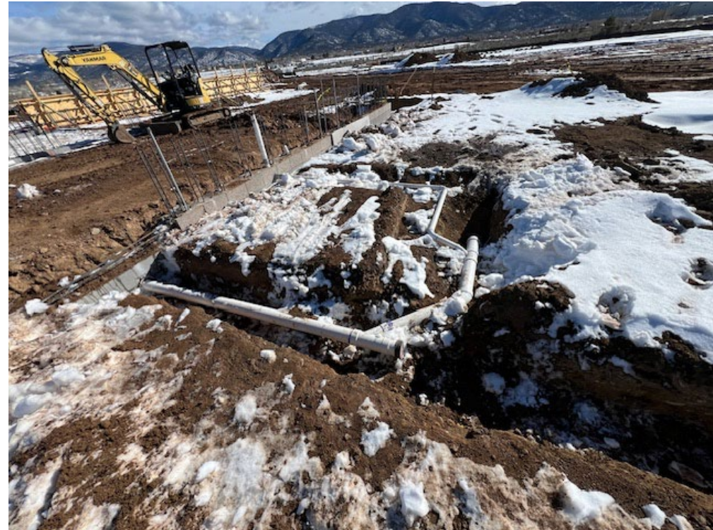
Plumbing and trench
