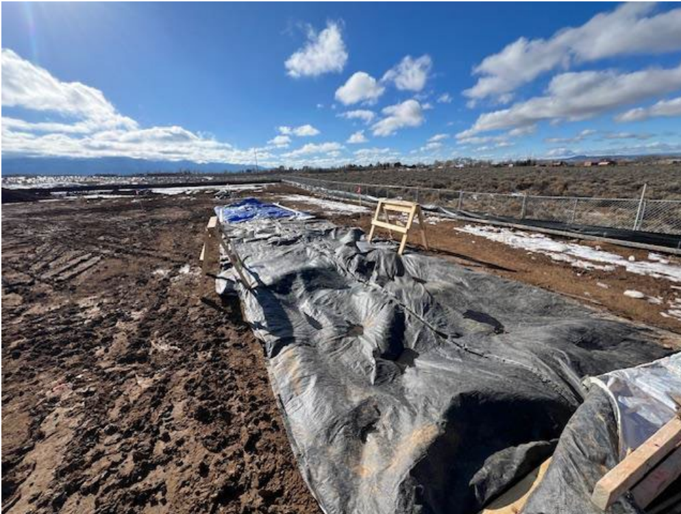
Fueling station island concrete protective sheets
