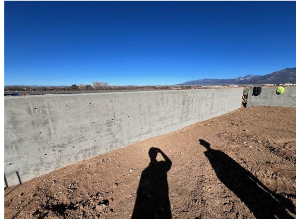
Concrete wall at north patio area
