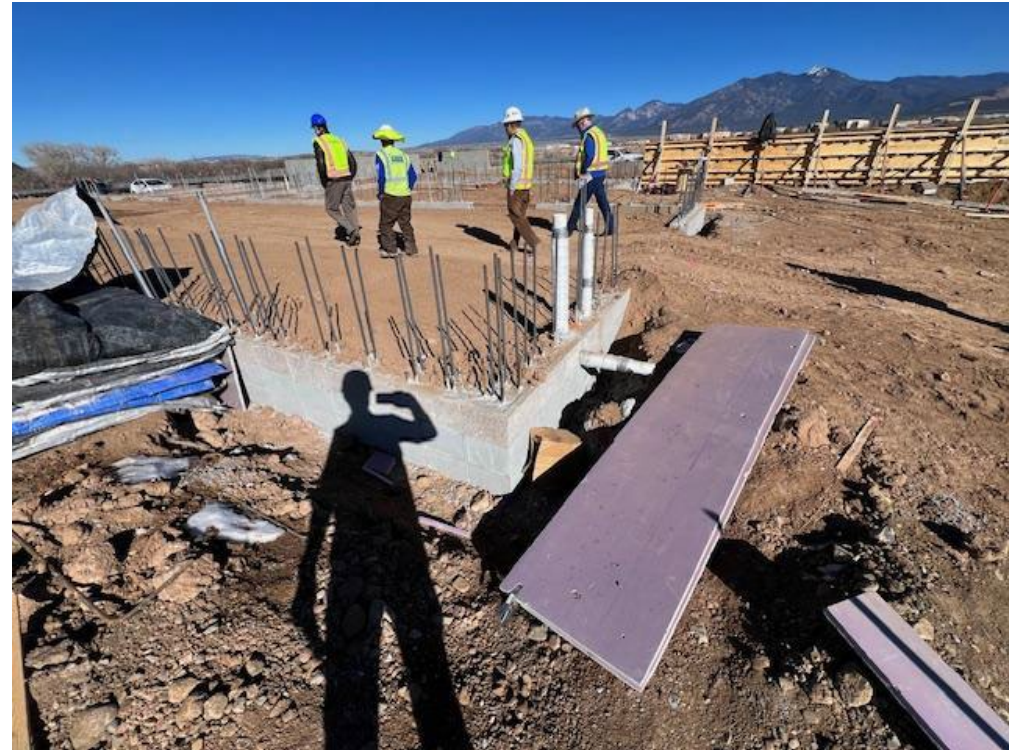
Plumbing and electrical rough-in
