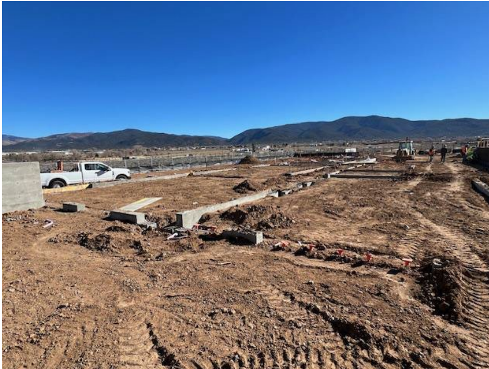
Masonry stem walls looking southeast
