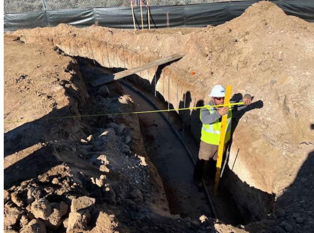
North retaining wall footing and rebar
