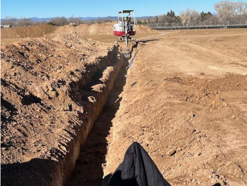
Secondary power conduit trench looking north
