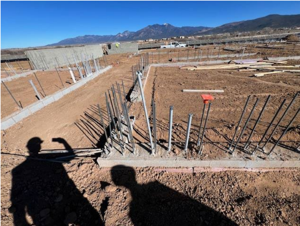
Plumbing and electrical rough-in
