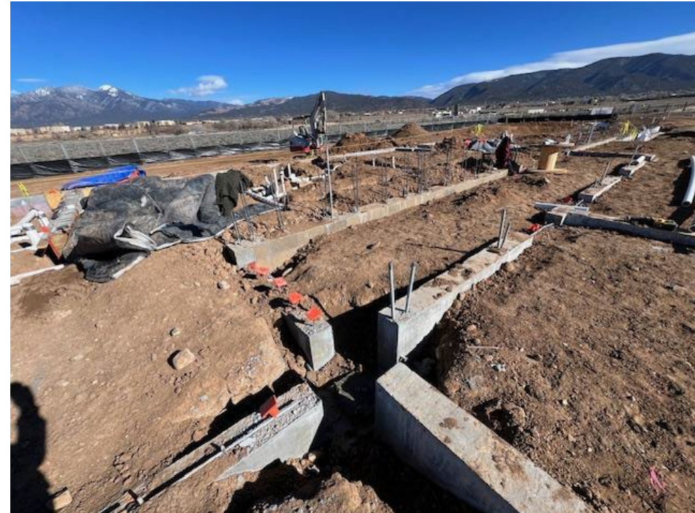
Concrete stem walls, rebar and electrical conduit
